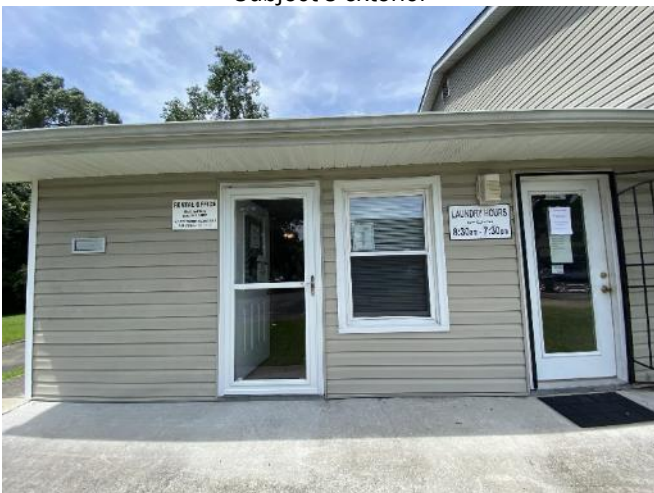
Management office exterior
